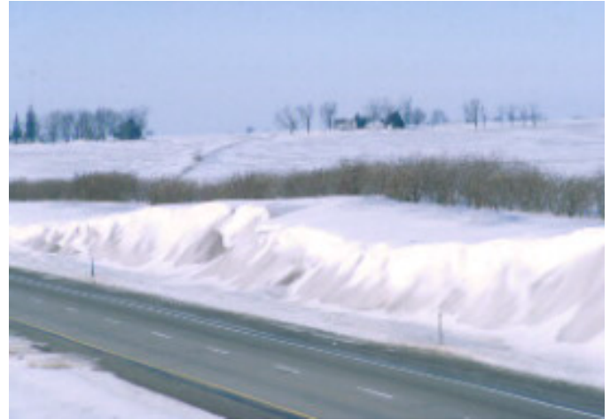
This roadside development project demonstrates the utility of native vegetation as a living snow fence, which prevents major snow drifting on the roadway.
